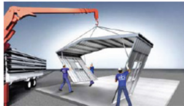
3 Abertura das paredes Opening of the walls
